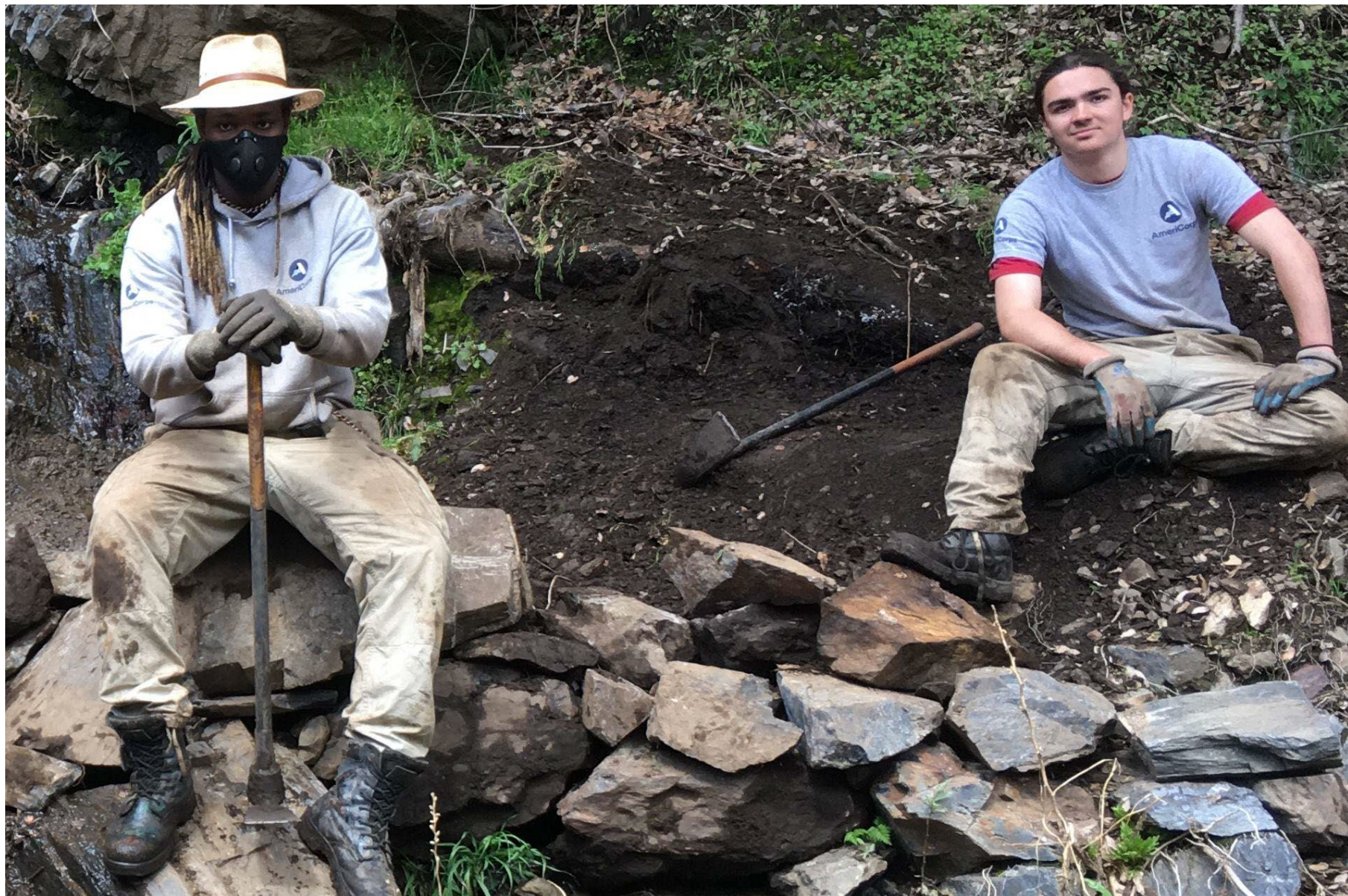
Americorps members sit on rock retaining wall they reconstructed on the Skelton Creek Trail.
