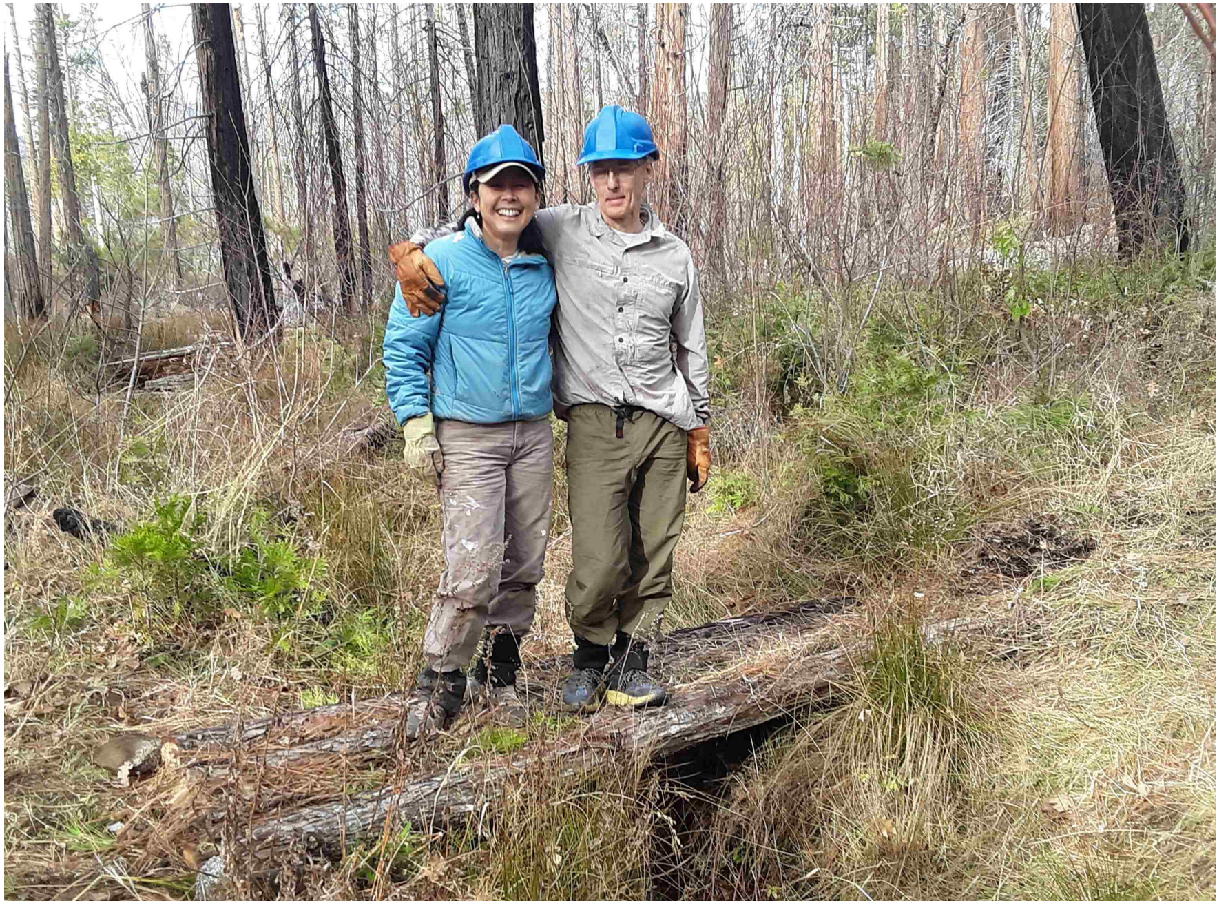
Theresa and Tom standing on the pedestrian bridge they just built on the Bishop Creek Trail
